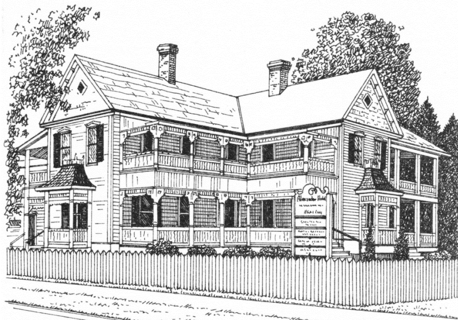
The Alexander Hotel Community Center
